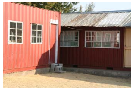
Above is a picture of the Maluti Seventh-day Adventist School in Lesotho. Fundraising will go towards building a new school. The building on the left is a steel storage container with windows and doors cut out.
